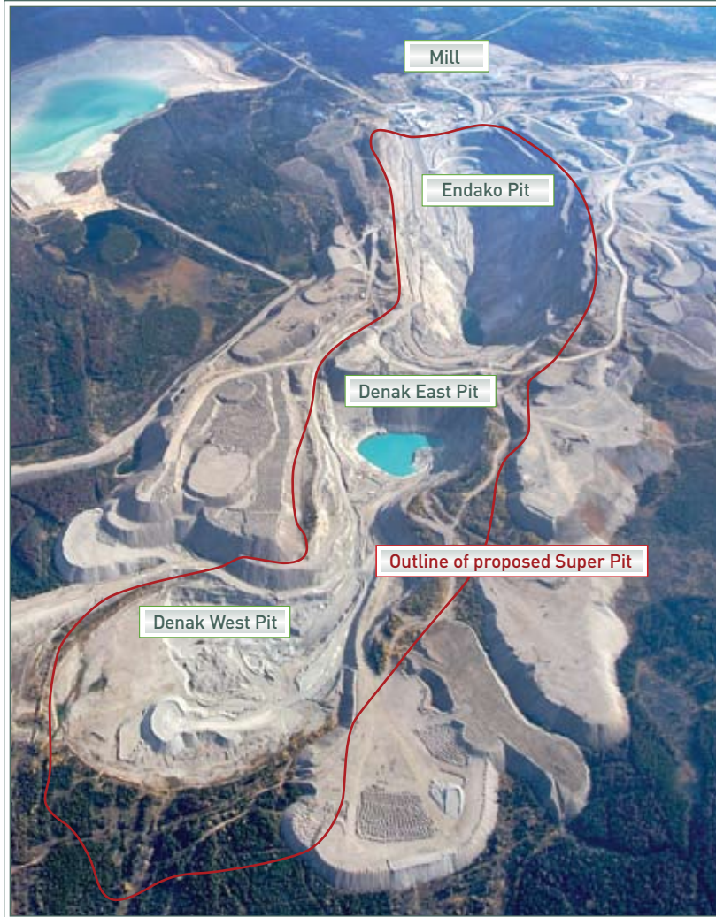
Aerial view of Endako Mine
