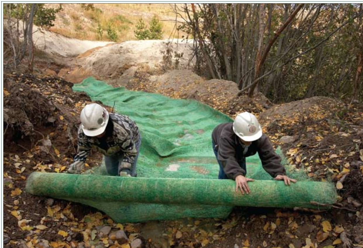
Erosion protection activity at Endako
