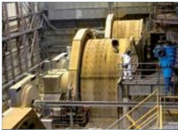
Grinding operations in mill at the Thompson Creek Mine
