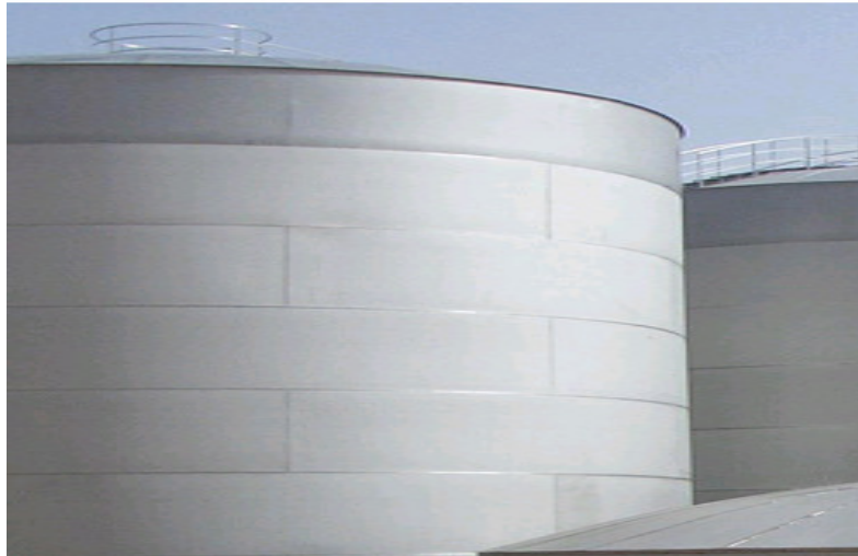
Lean duplex stainless steel containing about 0.3% molybdenum has started to take the place of molybdenum-free austenitic 304 stainless in the manufacture of storage tanks.
