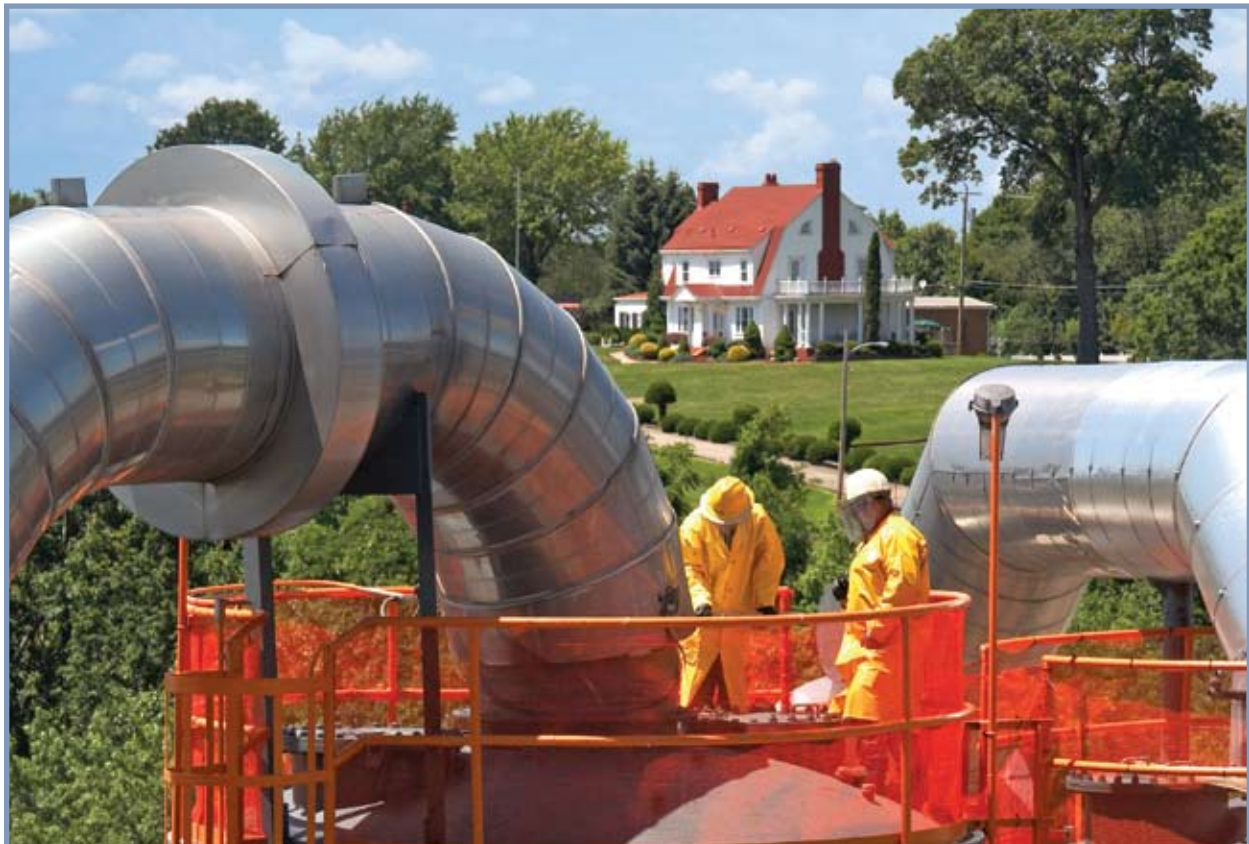
Servicing pollution control equipment at the Langeloth Metallurgical Facility
